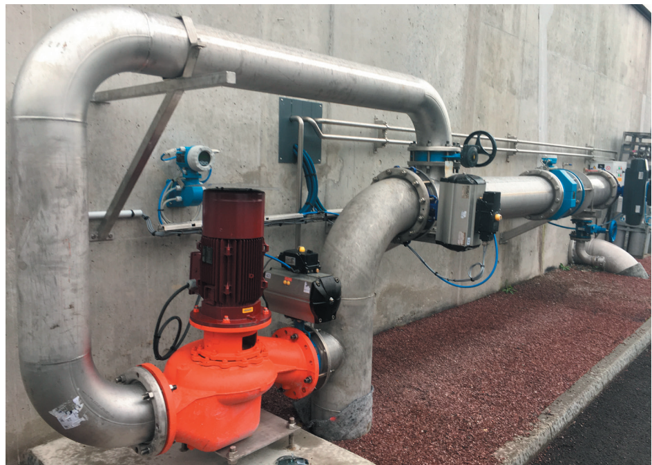
Figure 8. Pump as turbine in REDAWN pilot plant
