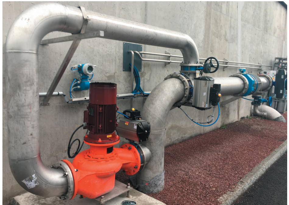
Figure 8. Pump as turbine in REDAWN pilot plant
